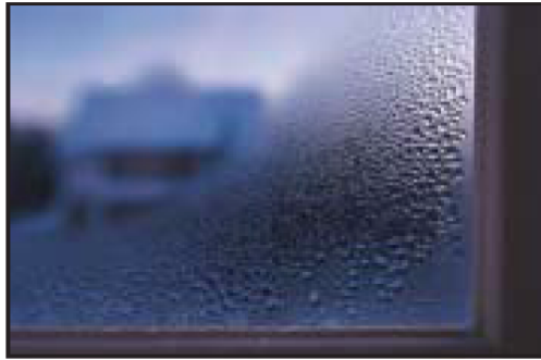
Condensation on the inside of a windowpane.
